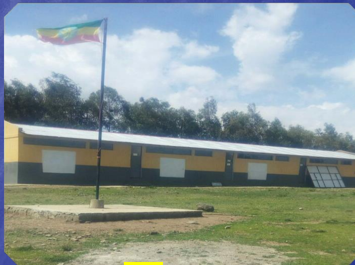
High School at Sodo Woreda
